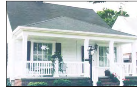
The remodeled home shown features Plantation Square columns with Architectural capitals and bases. It also utilizes Plantation style railings and matching newel posts.
