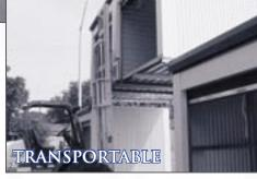
The doors and trim are available in 22 pre-finished colors. The roofs are sloped at 1/4:12 inch, and have leak proof screw downs. The roof can withstand 50 pound snow load and a 125 psf floor load. Windloads up to 130 mph can be obtained with simple tie downs.
